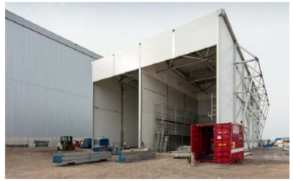
Temporary coating hall at Maasvlakte 2
