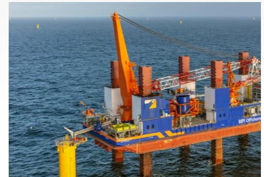
TP-less Monopiles for Hollandse Kust Noord
