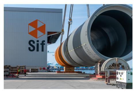
Picture: load-out monopiles for Dogger bank
