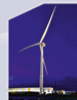
November Commissioning Haliade-X on Sif terminal
