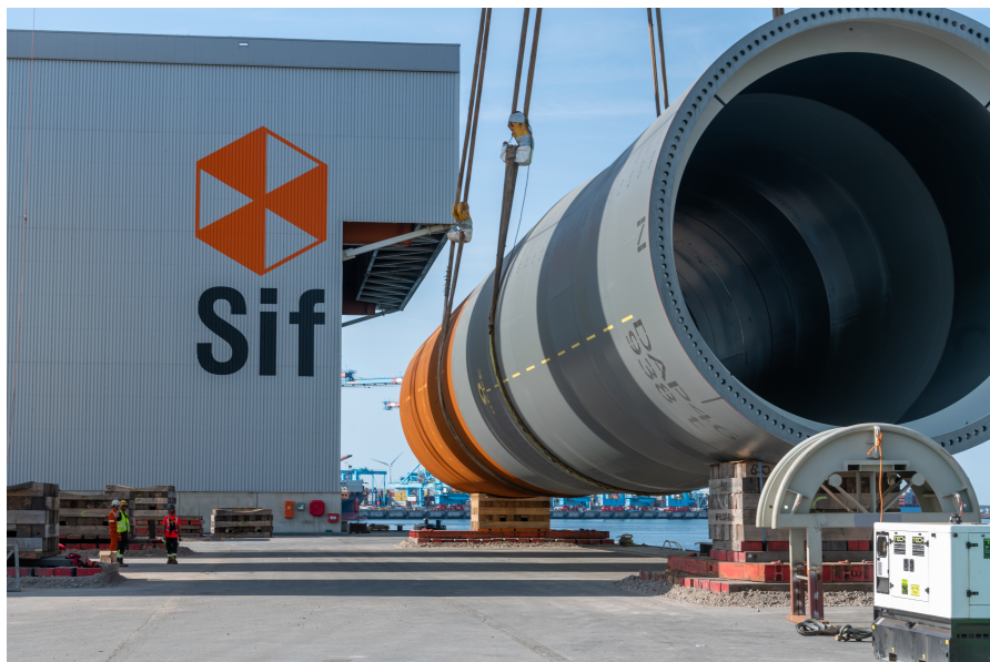
Loadout of monopiles for Dogger bank
