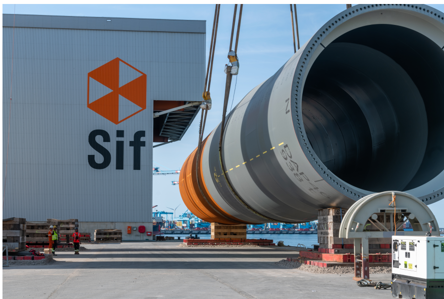
Loadout of monopiles for Dogger bank
