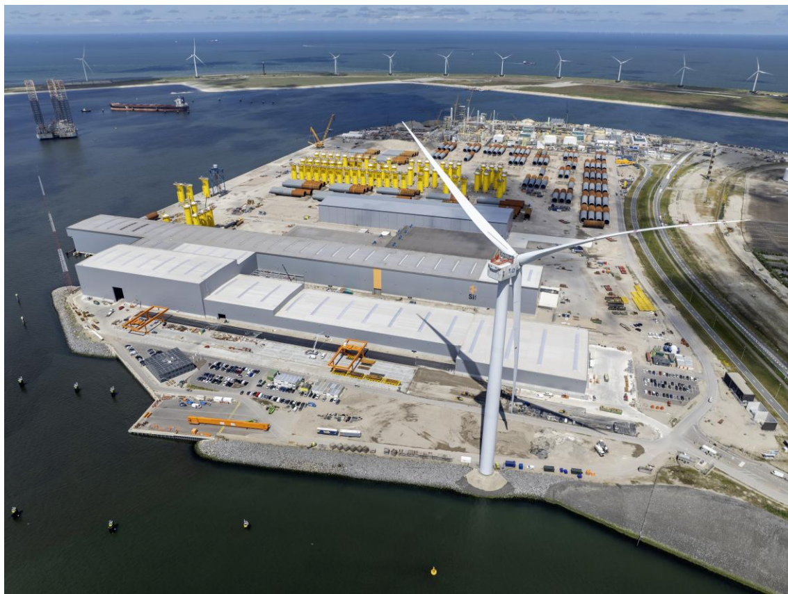
Expanded manufacturing facilities at Maasvlakte 2, Rotterdam. Situation in July 2024
